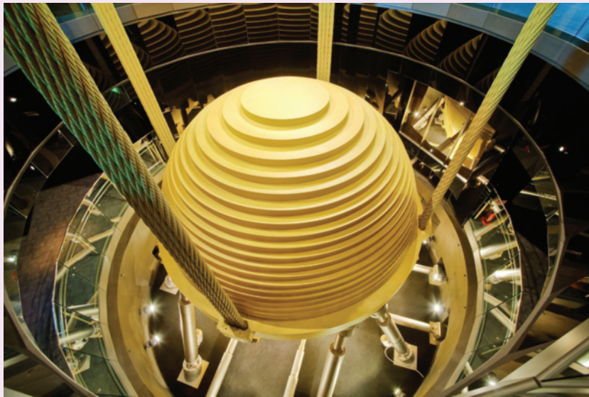
■ Figure 14.77 The Taipei 101 damper is designed to absorb energy in the event of an earthquake
