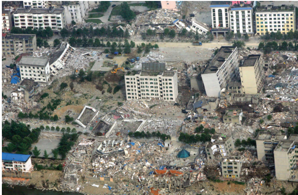
■ Figure 14.82 Resonance may be one reason why some buildings collapse in an earthquake
