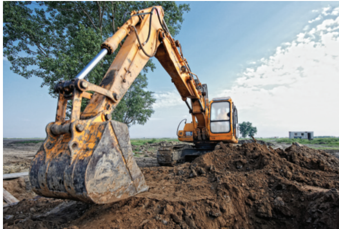
■ Figure 14.52 Hydraulic machinery is used in this excavator
